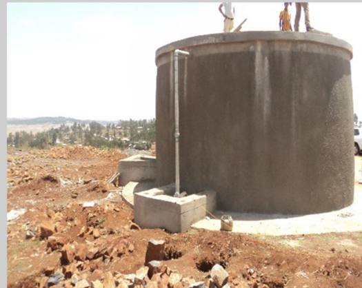
Proper civil work execution using the BCBT
